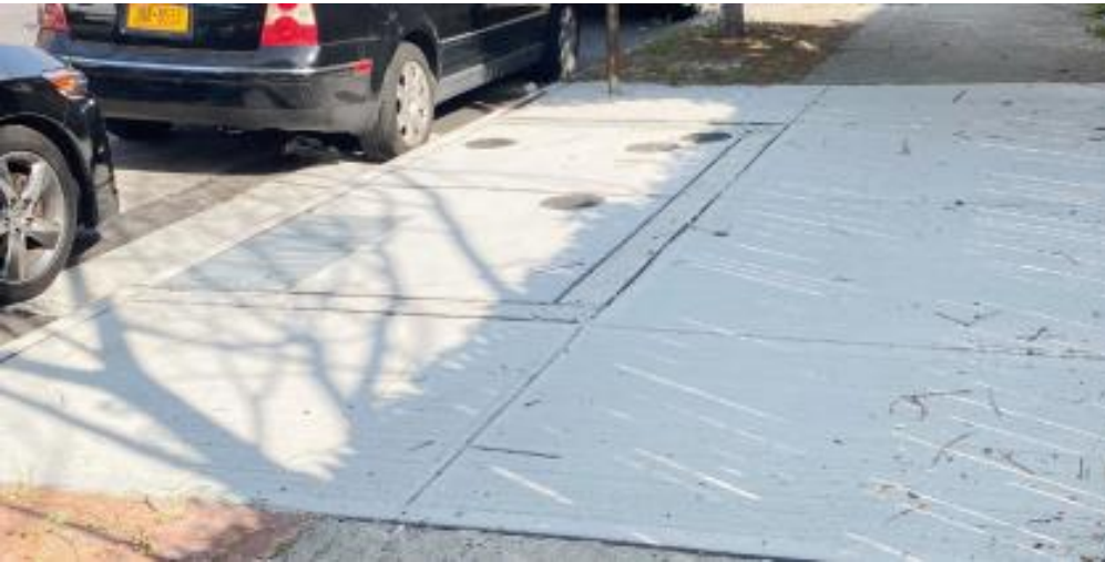
Infiltration Basin with Concrete Top
